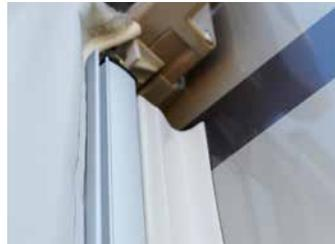
The mast profiles are fitted with rubber seals to prevent scratching and to make the area entirely waterproof. The height can easily be adjusted.
